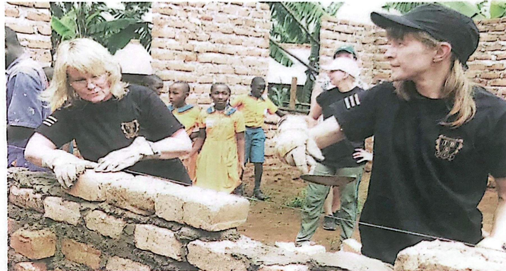
Burman and a colleague building a dormitory block in Mbarara recently. Photo by Abdulkarim Ssengendo
