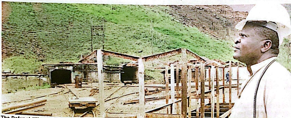
The Defunct Kilembe mines in Kasese. M2Cobalt company has expressed interest in re-developing Kilembe Mines
