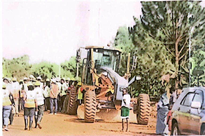
Government officials including Works and Transport minister Gen Katumba Wamala inspect works on Nakawuka-Kasanje-Mpigi Road in January. PHOTO/COURTESY OF MOWT X HANDLE
