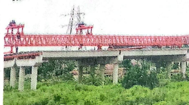
A section of the Kampala-Entebbe express highway in Ruwasa
