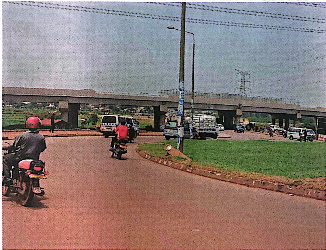
Heavy-loaded trucks and trailers are not expected to use the Entebbe Expressway
