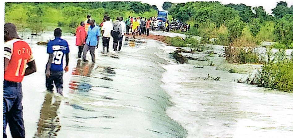
Residents crossing the submerged Alito bridge. In the background are stranded passengers after a bus failed to cross the bridge. Photos by Emmanuel Alomu
