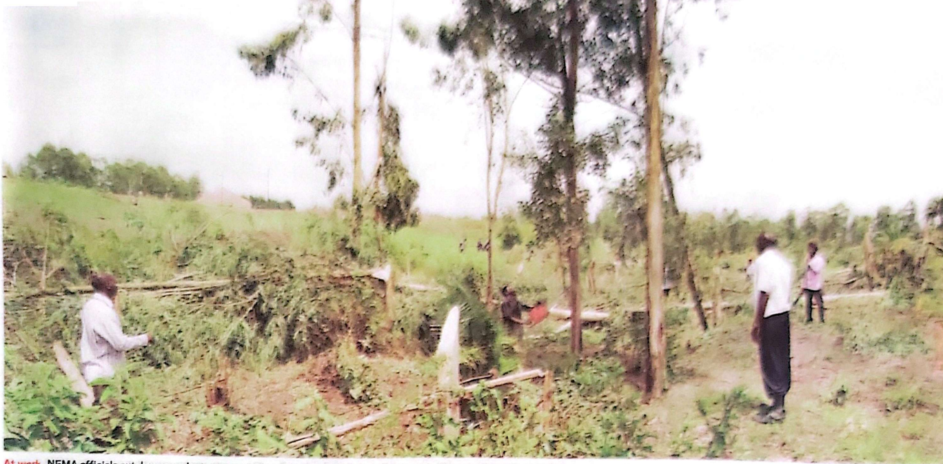
At work. NEMA officials cut down eucalyptus trees at River Rwizi banks in Bubare Sub-county, Mbarara District last week. PHOTO BY FELIX AINEBYOONA
