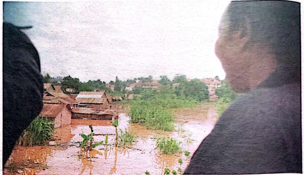
Submerged. Flooded houses at Kigowa Village, Kalinabiri One and Two on the Norther Bypass on Sunday.
