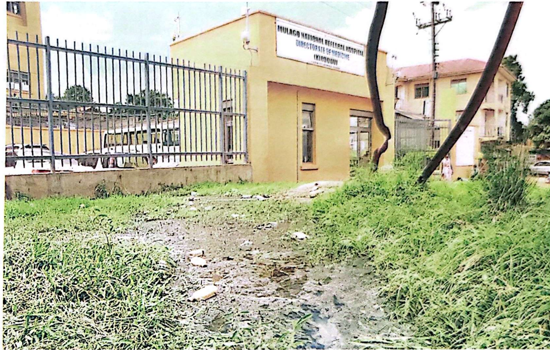
Challenge. An overflow of sewage at Kiruddu hospital yesterday. PHOTO BY ALEX ESAGALA
