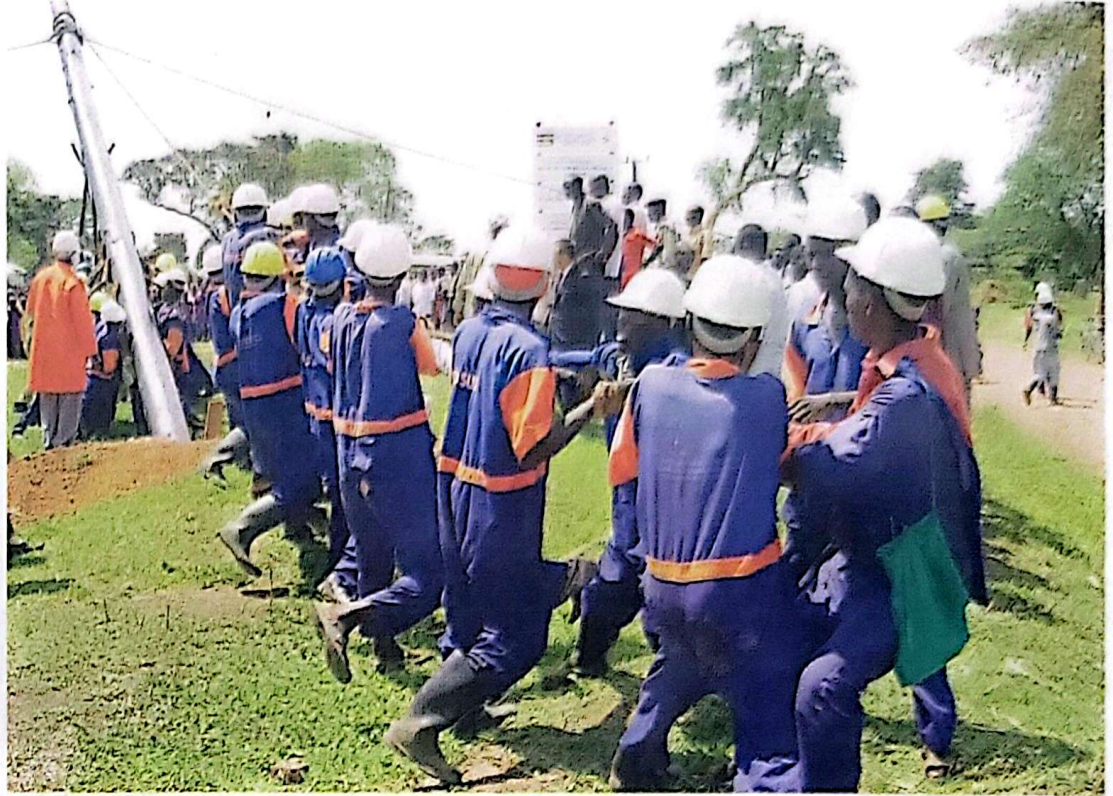
Workers erecting an electric pole during the commissioning of the second phase of rural electrification project at Nabitende, Iganga district in October 2009
