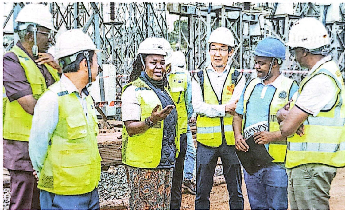
Energy minister Ruth Nankabirwa (centre) during a tour of the Kampala Metropolitan Transmission System Improvement Project at the Maya Sub-station in Mpigi District. PHOTO/GEOFREY MUTUMBA
