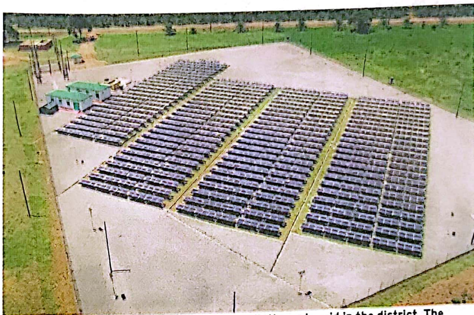
A solar plant in Kalangala that supplies power to the main grid in the district. The Government is investing in alternative energy sources to boost the national grid
