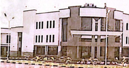
Uganda House Abuja as of December 2025.
