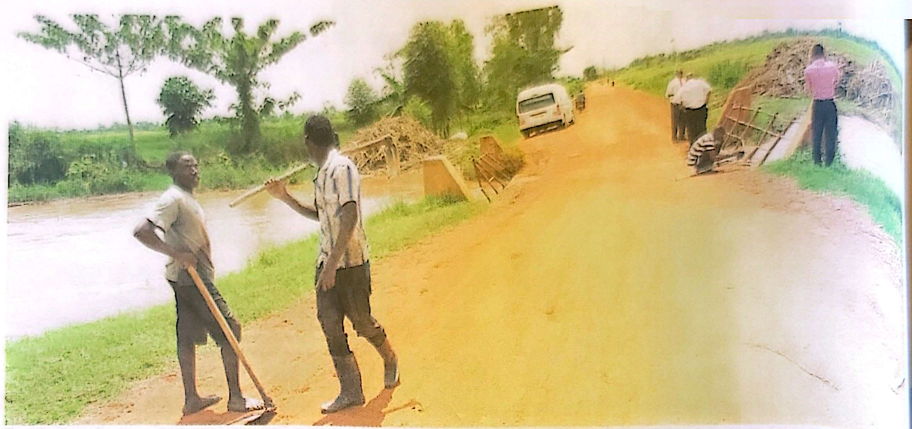
Residents using a partially flooded bridge in Doho parish, Butaleja. Photo by George Bitu
