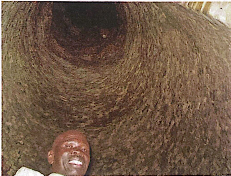
A DRB miner stands in the now demolished anti-pollution chimney in Jinja. Photos by George Bitu
