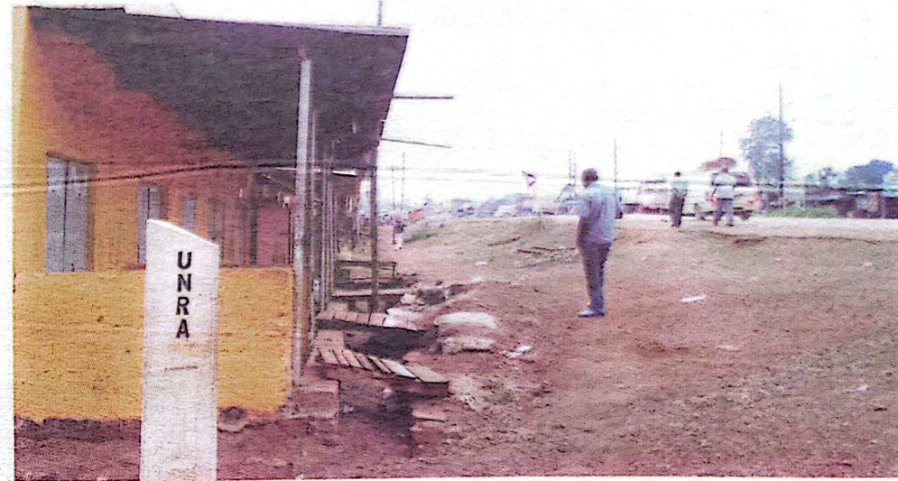
Illegal. Some of the structures in Buwama Town on the Kampala-Masaka highway that were constructed in a road reserve.
