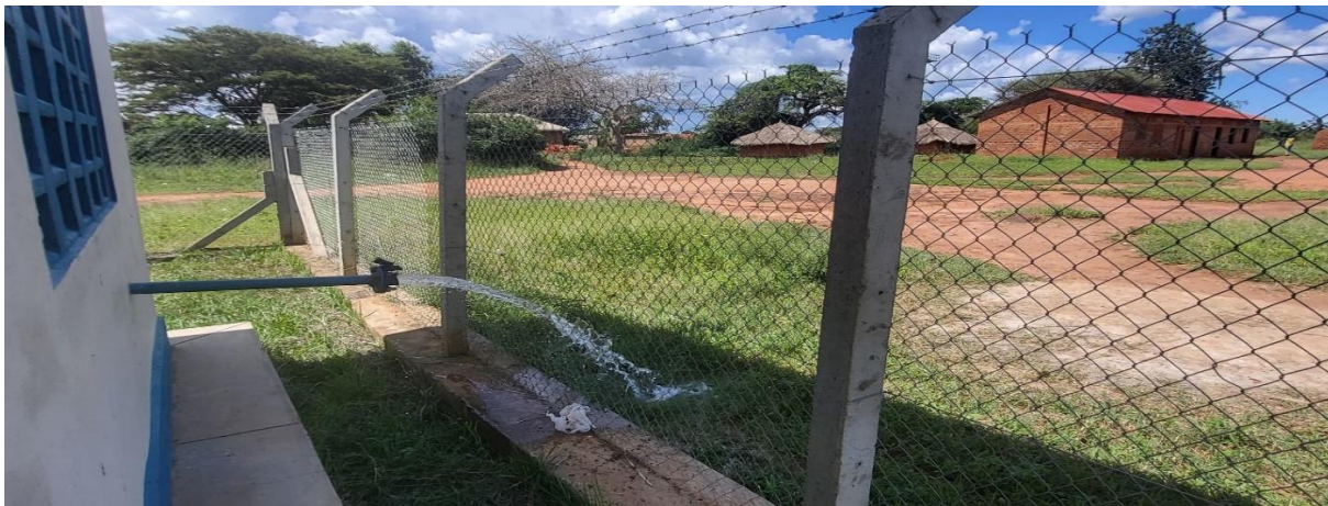
Figure 3 showing water discharge of the well
