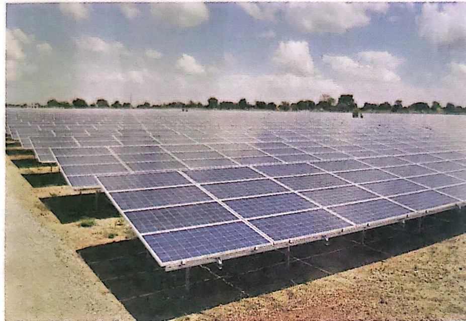
New. Soroti PV Solar farm. The Tororo Solar North plant will generate 10 megawatts. FILE PHOTO
