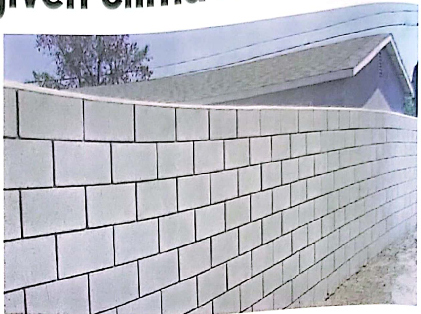
Stabilised blocks do not require firing and so no firewood
