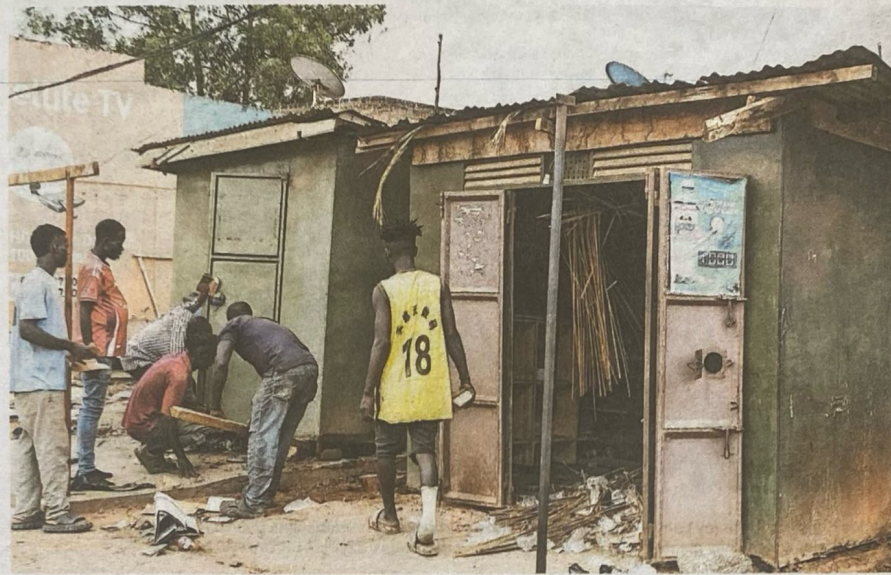
Men remove kiosks on the Arua-Nebbi road. Dozens of traders who once depended on small stalls were pushed out in recent evictions aimed at decongesting the cities and enforcing the trade order. PHOTO/FELIX WAROM OKELLO
