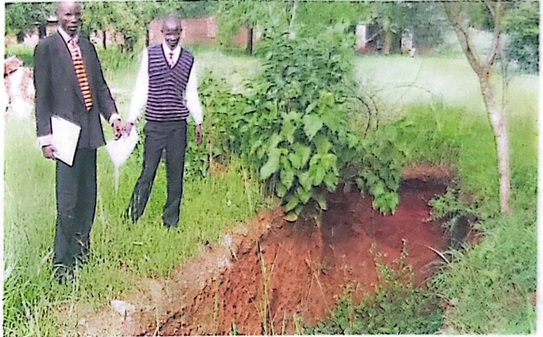
Adaku (wearing jacket) and Opalto at the excavation site of the five-stance toilet at the school in Arua. Photos by Robert Ariaka
