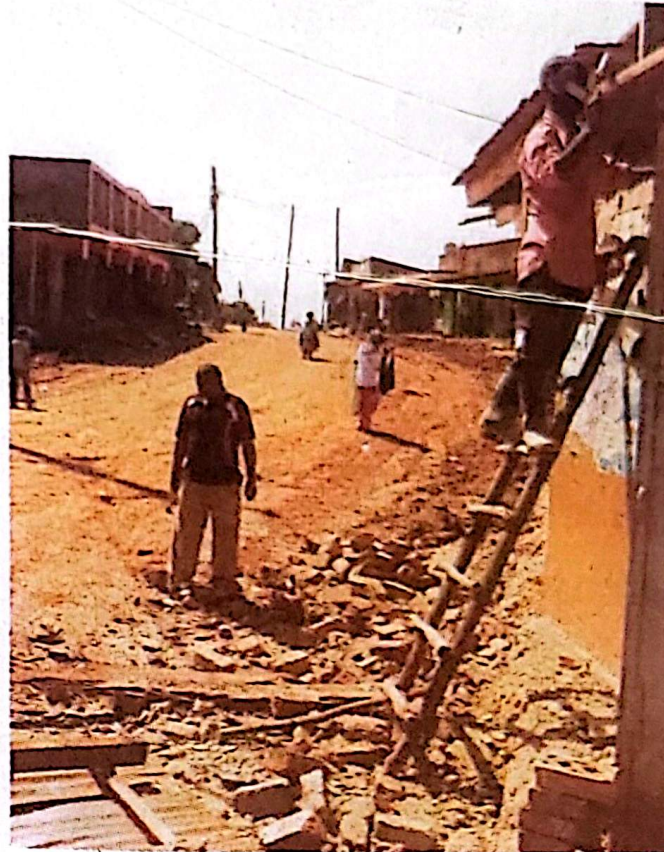
Paving way. A resident demolishes part of his shop in Kanyanaya Village, Makindye Ssabagabo to pave way for the expansion of a road.
