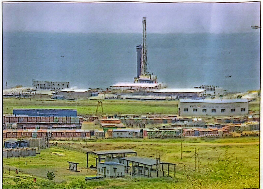
The facility at the Kingfisher oil field in Buhuka Parish, Kikuube district, where Uganda is advancing oil development activities as discussions with DR Congo on joint cross-border exploration gain momentum
