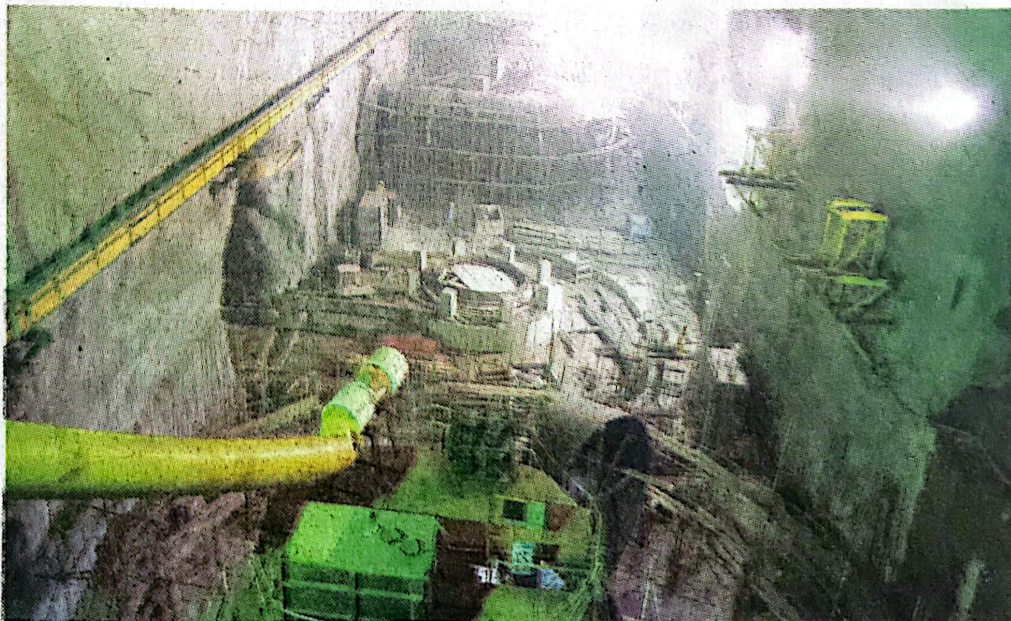
Progress. The power house at Karuma Hydro Power plant under construction. PHOTO BY TOBBIAS JOLLY OWINY
