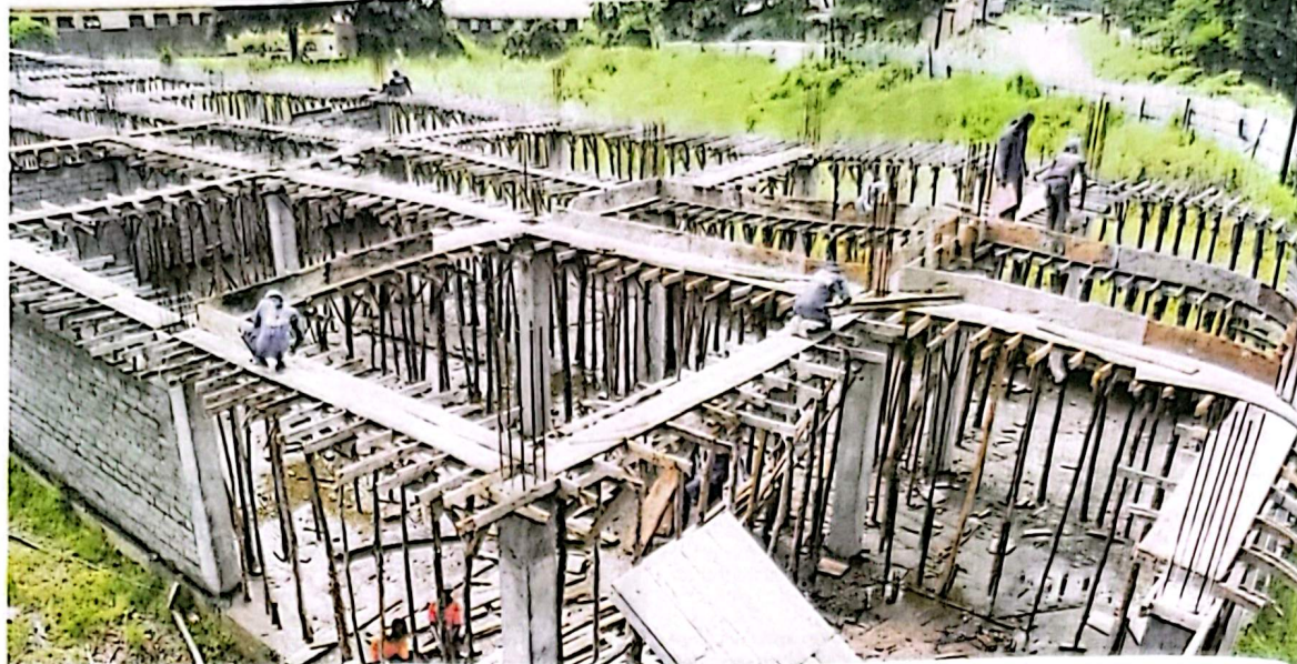
Workers at a construction site. Instead of flat fines, the law pegs penalties to the size of the building, making non-compliance more expensive. PHOTO/FILE
