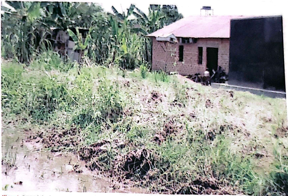
Illegal. One of the houses that have been constructed in a wetland in Adjumani Town. PHOTO BY FELIX WAROM OKELLO.
