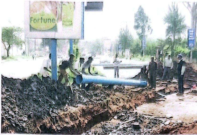
Workers of NWSC installing water pipes along Jinja Road at Lugogo in Kampala. People still find difficulties getting safe water despite increased access to piped water
