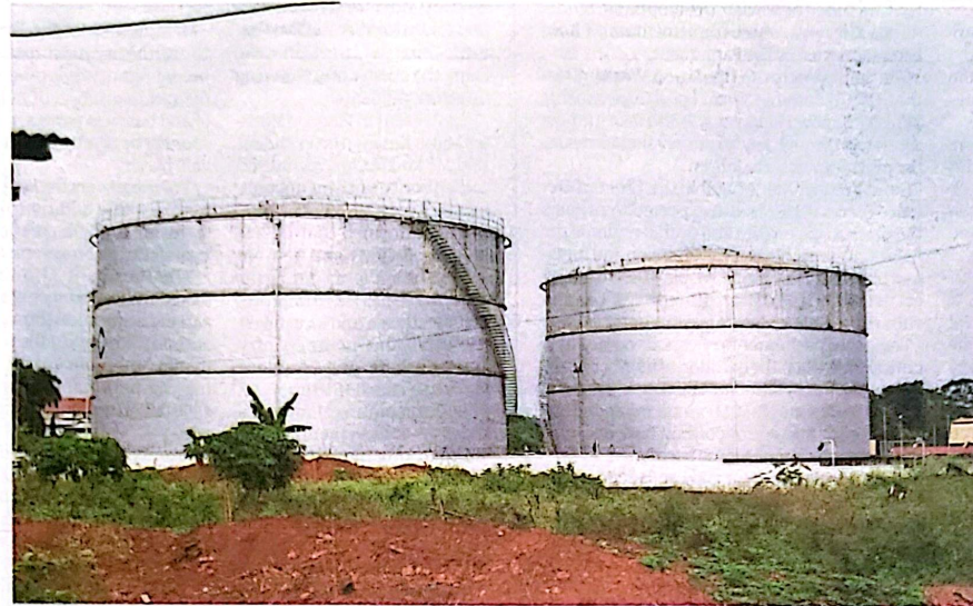
A section of fuel reserve tanks operated by the Uganda National Oil Company in Jinja City. PHOTO/FILE
