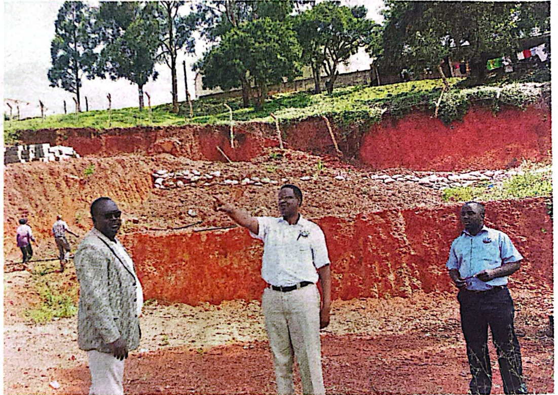
Samuel Apedel (left) and Eng. Alex Gisagara (centre) inspecting Muyenga Tank Hill recently. In the background is a water reservoir. Photo by Juliet Kasirye
