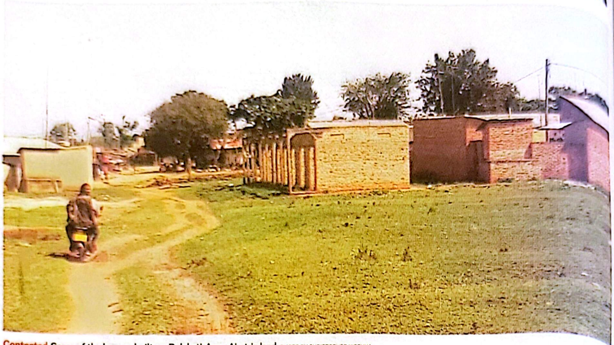
Contested. Some of the houses built on Bulakati Army Airstrip land. PHOTO BY CHRISTOPHER KISEKKA
