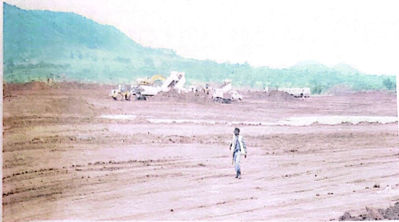
Kabaale Airport currently under construction in Hoima district. PHOTO BY ERONIE KAMUKAMA
