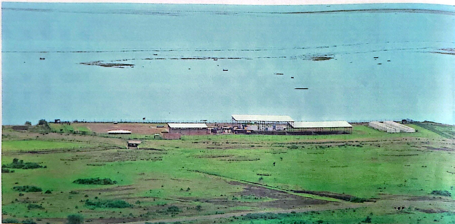
Occupied. An oil field operated by Cnooc on the shores of Lake Albert in Holma District. Preliminary estimates by the Petroleum Authority show that around 75,000 cubic metres (m 3 ) of water will be drawn from Lake Albert.
