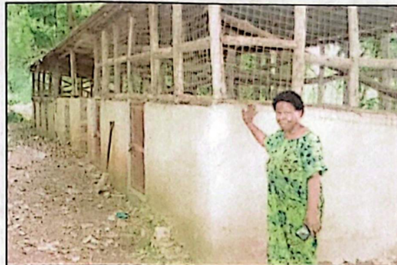
The structures housing the piggery project. The farm has 50 pigs
