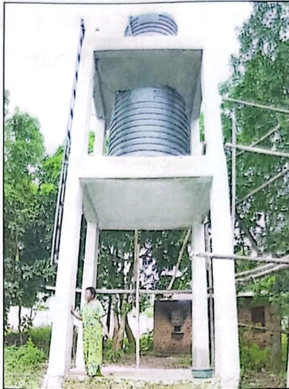
Sanyu pumps underground water into these tanks for irrigation
