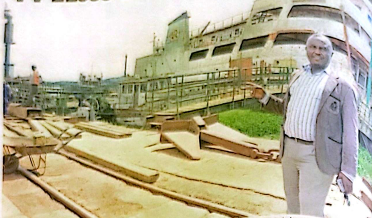
Renovation work going on at the Port Bell Pier. In the background, is one of the wagon ferries in need of repair
