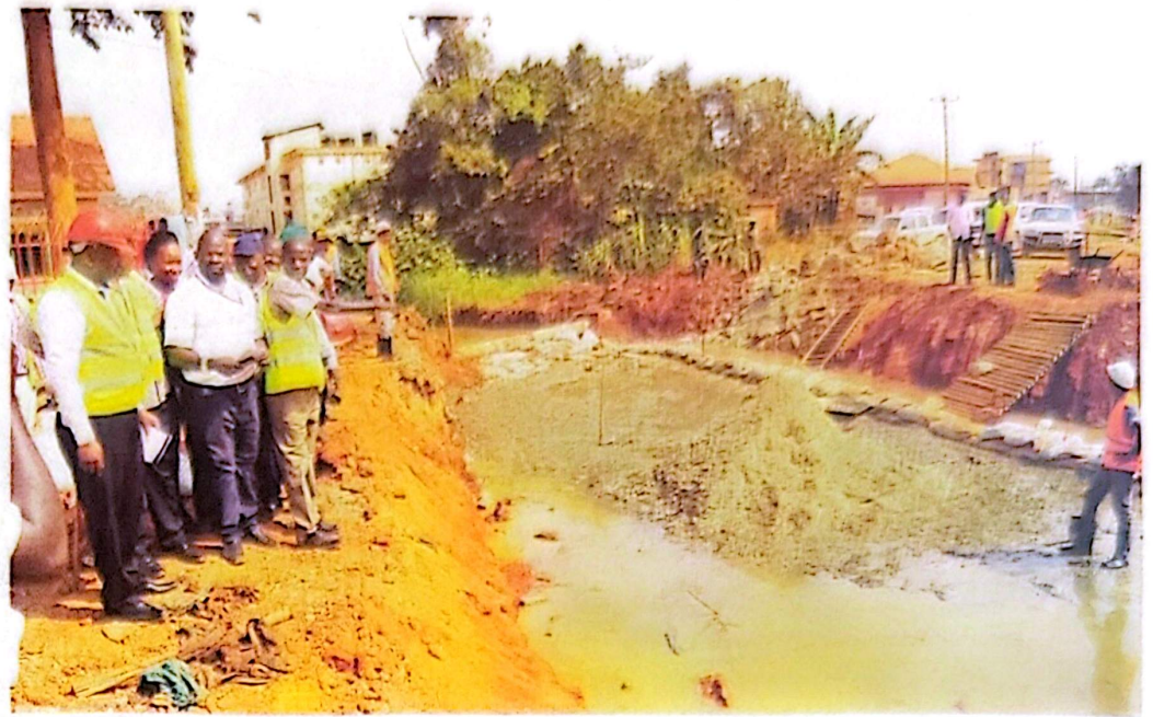
On the ground. Wakiso District officials and Works ministry engineers inspect ongoing works on Lufuka drainage channel along Mamasuba- Ndege Kitiko road in Wakiso District recently. PHOTO BY JOSEPH KIGGUNDU
