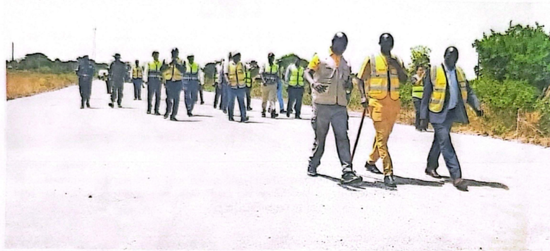
State minister for Transport Musa Eweru (left) and district leaders inspect a section of Koboko-Yumbe-Moyo Road, which is being tarmacked, at the weekend. PHOTO/ROBERT ELEMA
