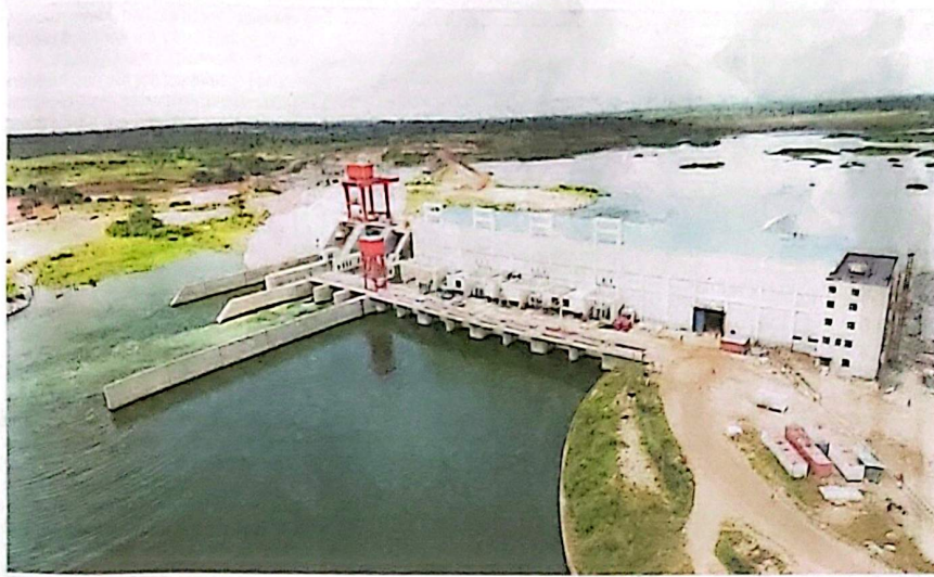
An aerial view of Isimba hydro electricity dam. According to UETCL's System Operations Data 2025 report, the stagnated increase in net electrical energy supplied from the plant to it was registered at 1.0 percent in 2025. PHOTO/FILE
