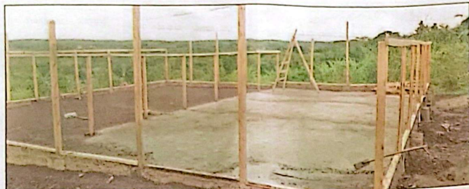
The co-operative is building a drying facility that will be powered by solar as one of efforts to ensure quality beans
