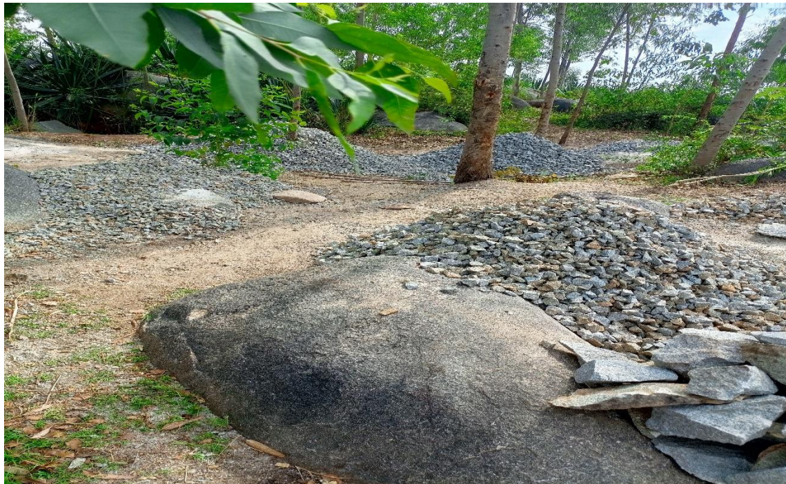
Figure: 4.2.6 Showing building materials inform of aggregates
