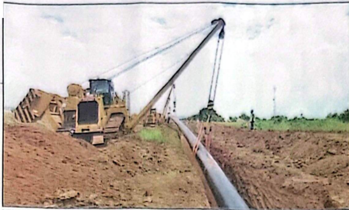
Lowering of pipes during the initial stages of the East African Crude Oil Pipeline project. The project is now left with only 15% of the works to be commissioned
