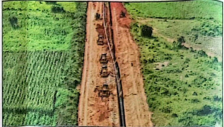
Ongoing works at the EACOP pump station one in Hoima district. The area marks the starting point of the EACOP on its journey to Tanga in Tanzania
