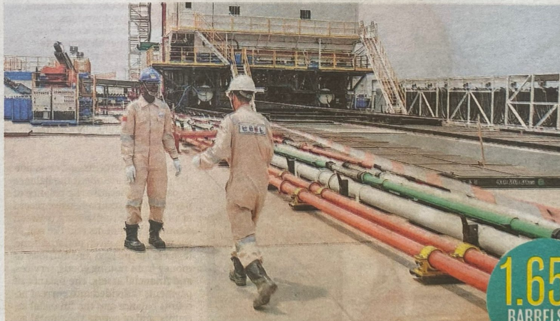
Workers at the Kingfisher oil field in Kikuube District on January 24, 2023. PHOTO/XINHUA
