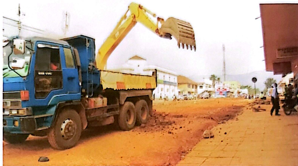
Construction. Road works on Republic Street Road in Mbale Municipality. World Bank officials accuse the municipality officials of delays. FILE PHOTO
