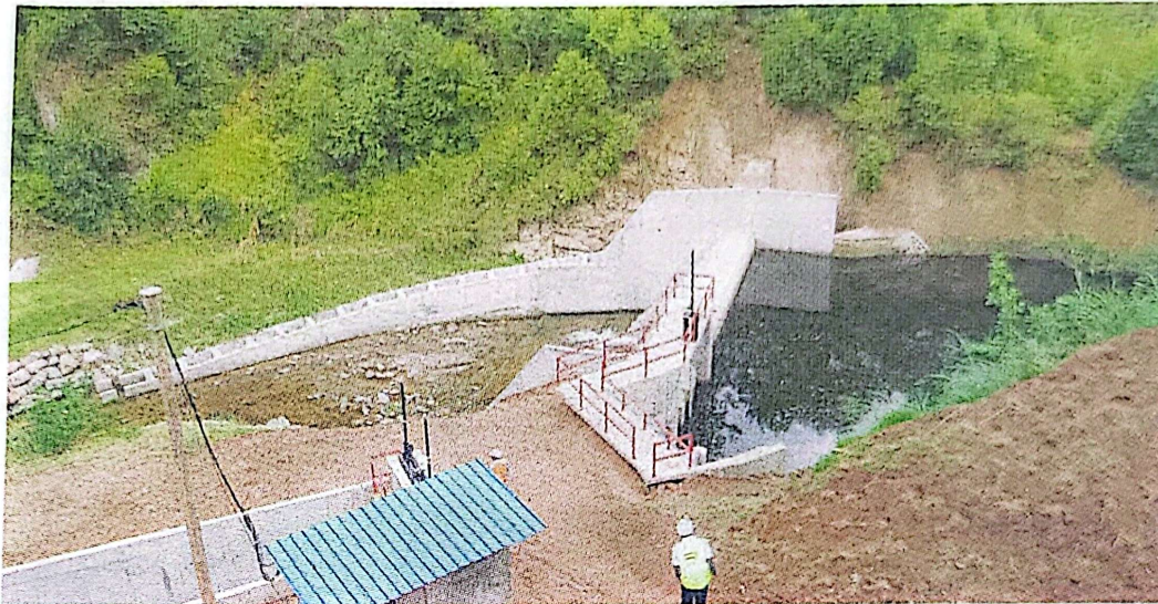
The Lubilia project that was completed recently. Photo by Benon Ojiambo
