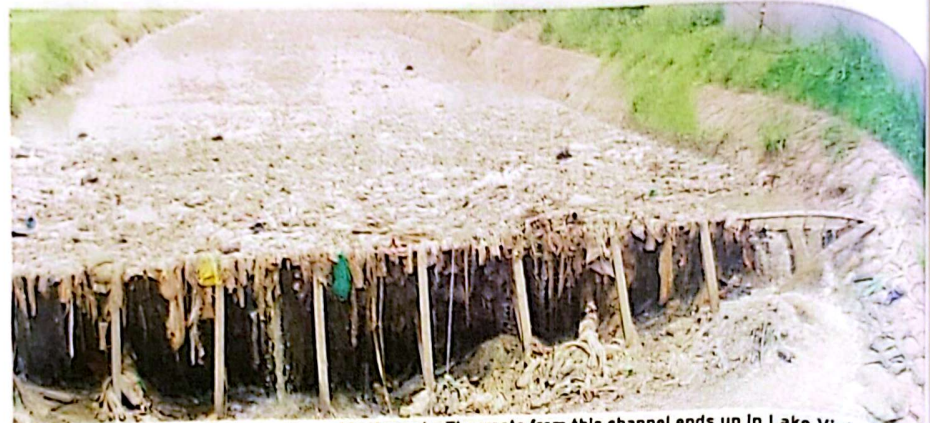
Polythene bags choking Nakivubo Channel in Kampala. The waste from this channel ends up in Lake Victoria
