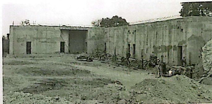
Bunker under Construction.
