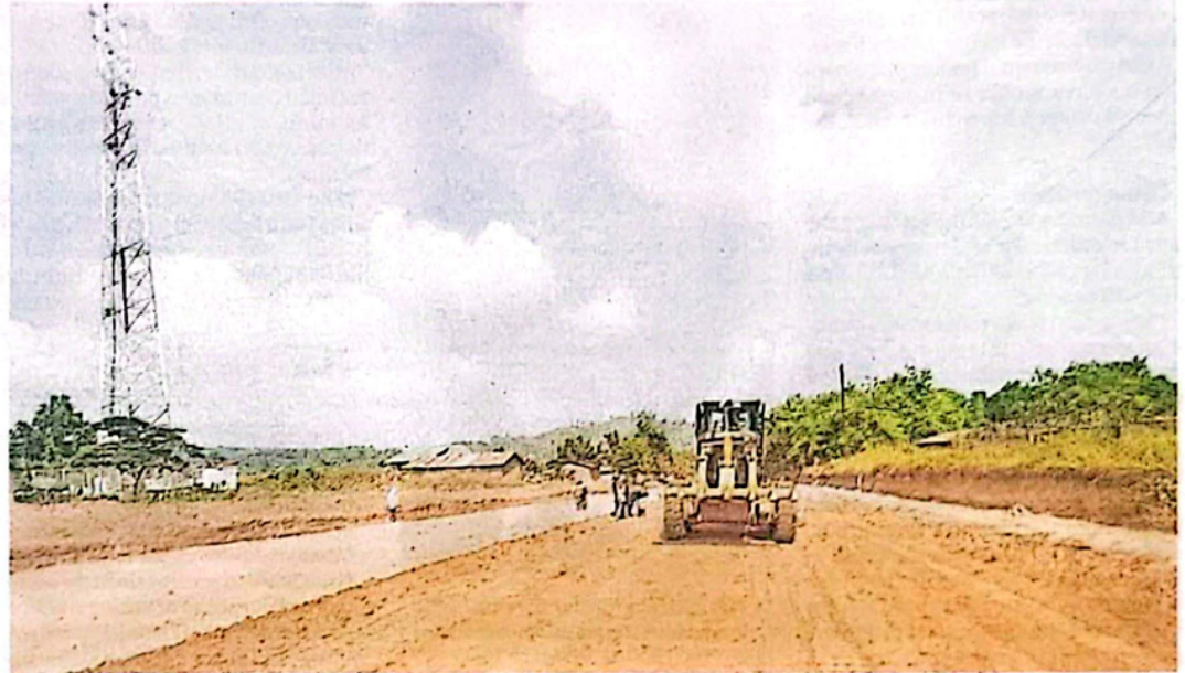
Workers prepare to lay asphalt on Kasindi-Beni road, an 80km stretch that links Uganda to Beni Town in DRC. PHOTO/ COURTESY
