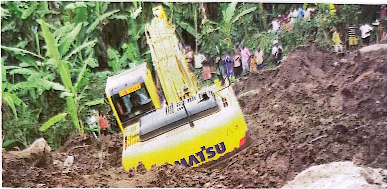
An excavator stuck in mud in Lusalanje Village, Masaba Sub-county in Sironko District. It was hired by police to search for missing people who were buried alive by mudslides.
