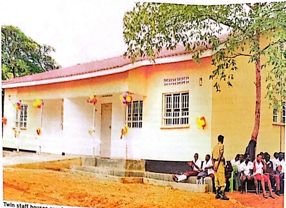
Twin staff houses constructed for Moroto High School by the Karamoja Affairs Ministry in 2016. Government has earmarked sh. 1 trillion for teachers' houses this year
