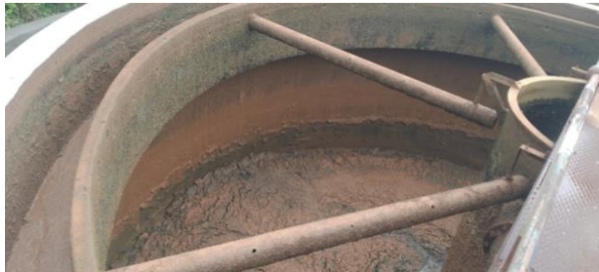
Figure 3.2: : Inside the clarifier sludge
