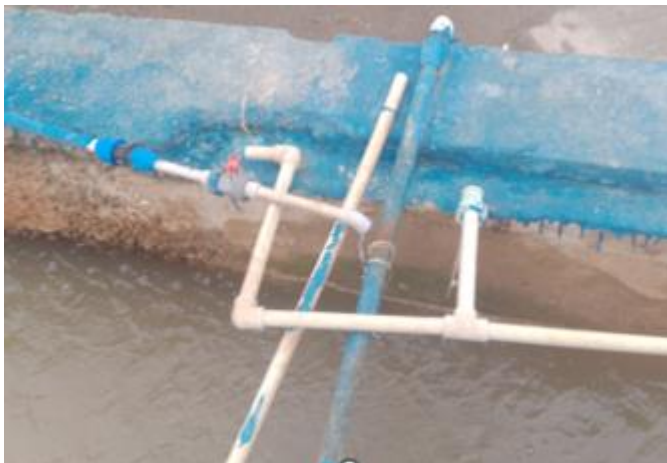
Figure 2.1 Showing alum solution being applied to raw water:
