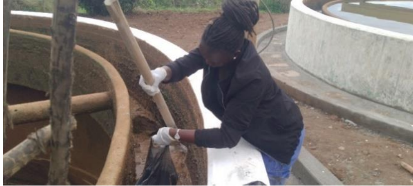
Figure 3.1: Outside clarifier sludge
