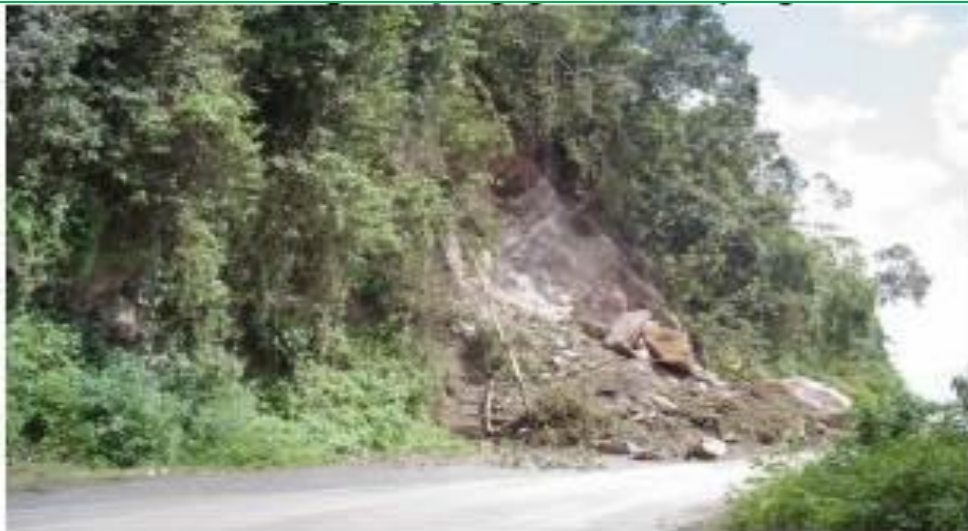
Photo 1: Landslides on Gikongoro-Cyangugu road in Nyungwe National Park (Rwanda) Source: GoR, MINITERE 2005. Initial Communication to the UNFCCC
